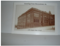
J. W. Cooper Building
